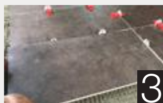
3 Place the other Tile over the other end of Tile Spacer
