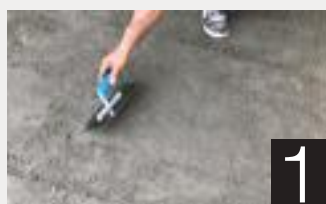
1 Apply Tile Glue / Cement
