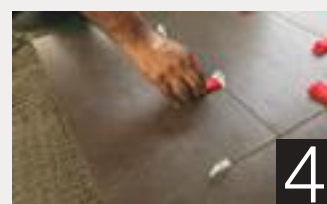
4 Insert Wedge into the Tile Spacer
